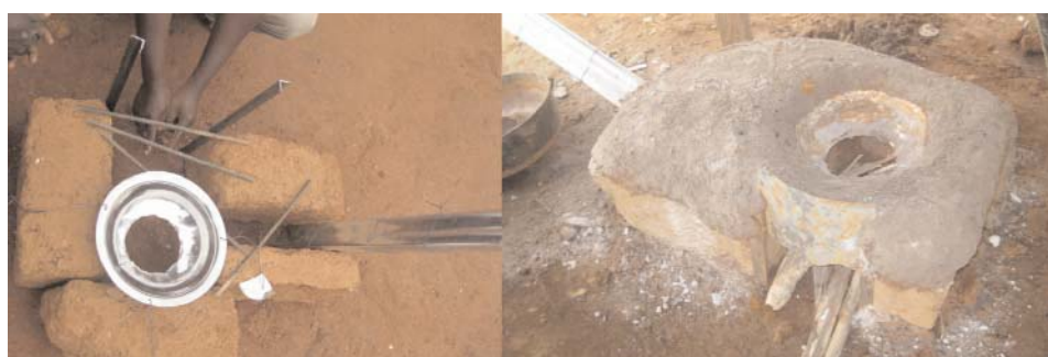
Construction of fuel efficient wood stove by DIN in Wula Ekumpuo
